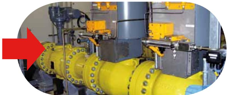
*HIPPS prevent over-pressurization by shutting down the source of the high pressure.*
