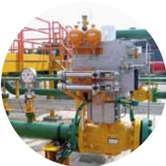
HIPPS with two Mokveld mechanical initiators protecting Shell Tutong metering station in Brunei.
